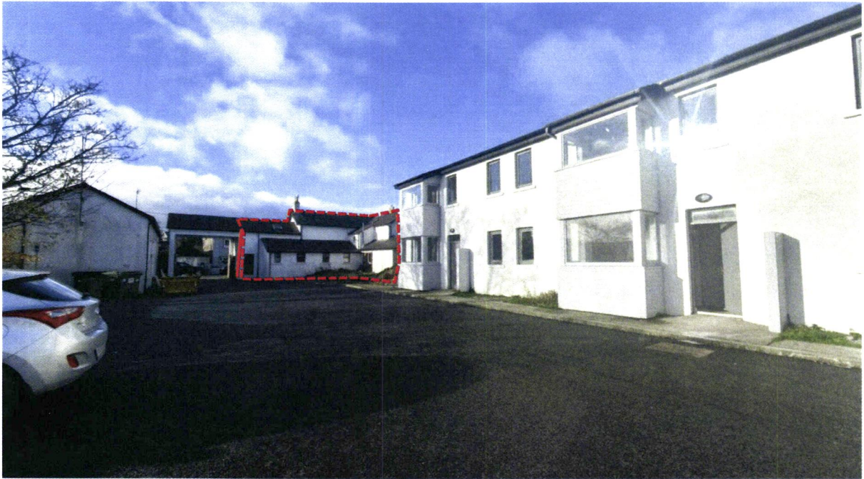
Reference Image 03: Rockingham House and Unit 3 (Rear)
